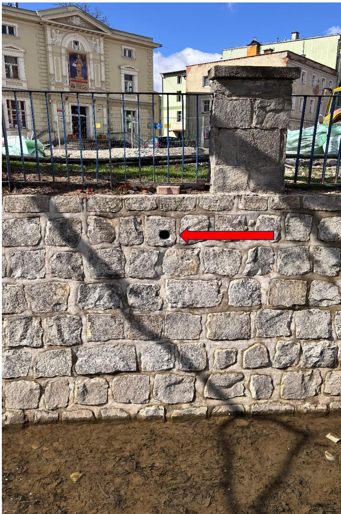
Phot.6. The red arrow indicates a nesting niche for birds made in the retaining wall (item no. 70).
