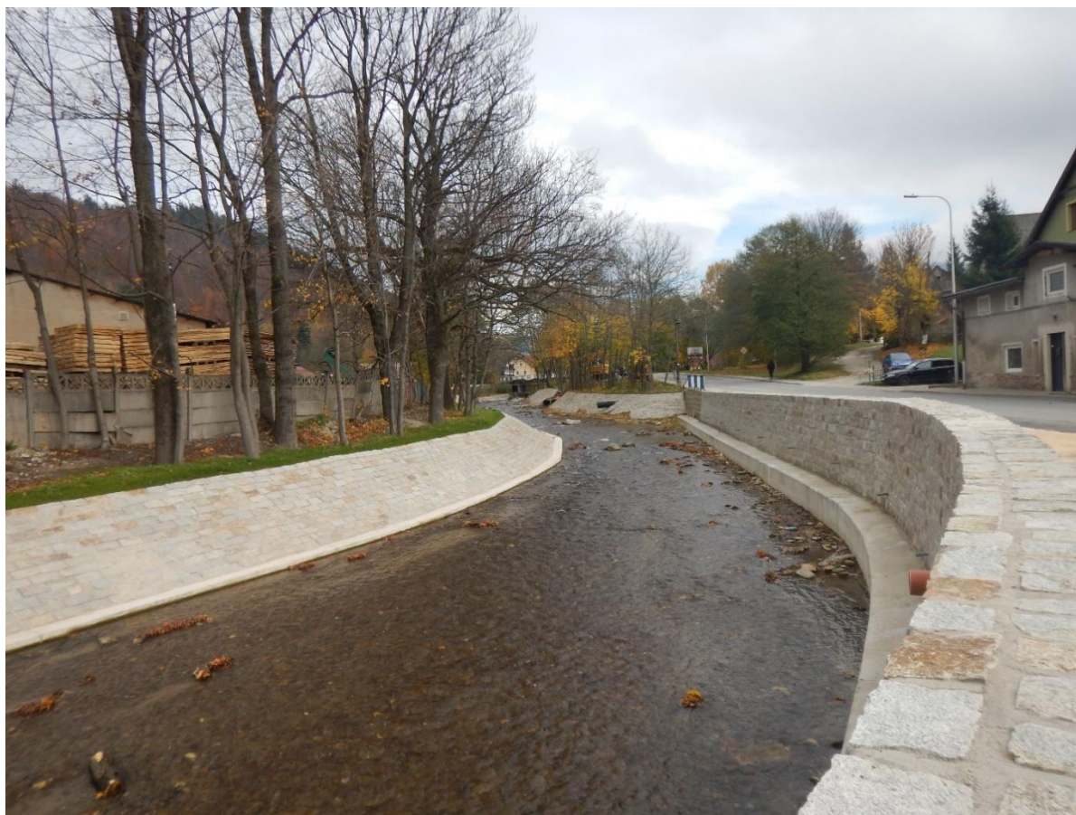
Phot. 23. Stronie Śląskie – view of the reconstructed retaining wall and slope revetment.
