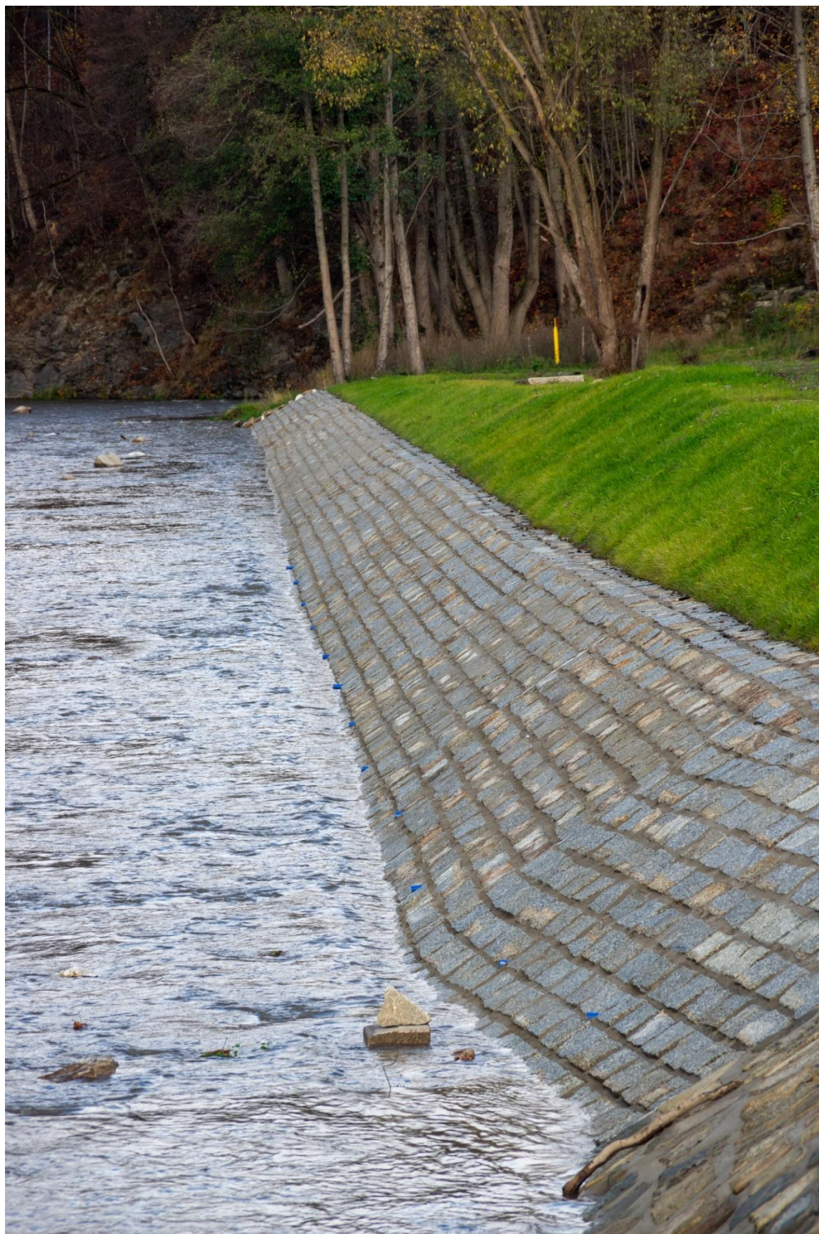
Phot. 25. Łądek Zdrój – reconstructed slope revetments.
