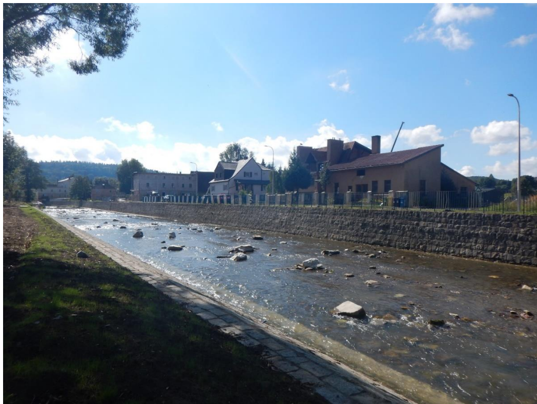
Phot. 11. Microhabitats for fish in the riverbed made after completed construction works (item no. 72).
