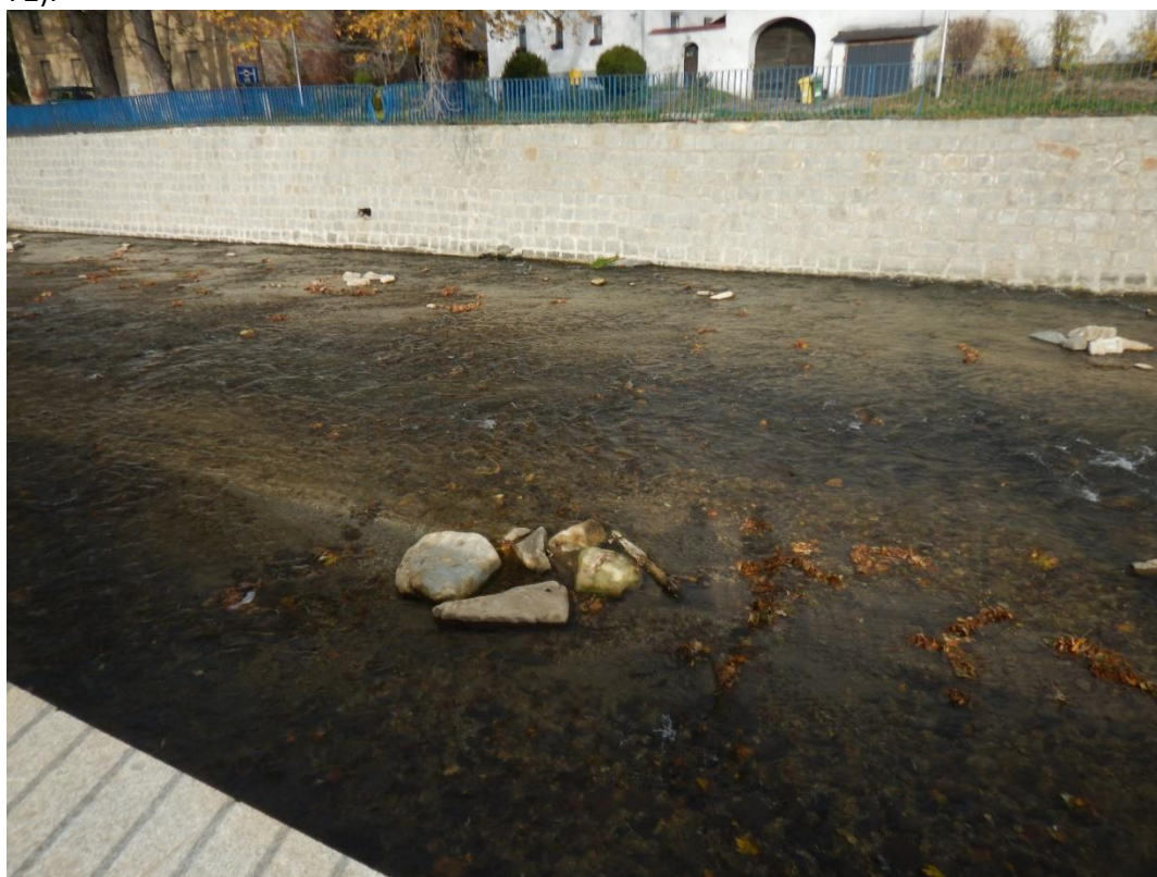
Phot. 12. Microhabitats for fish in the riverbed made after completed construction works (item no. 72).
